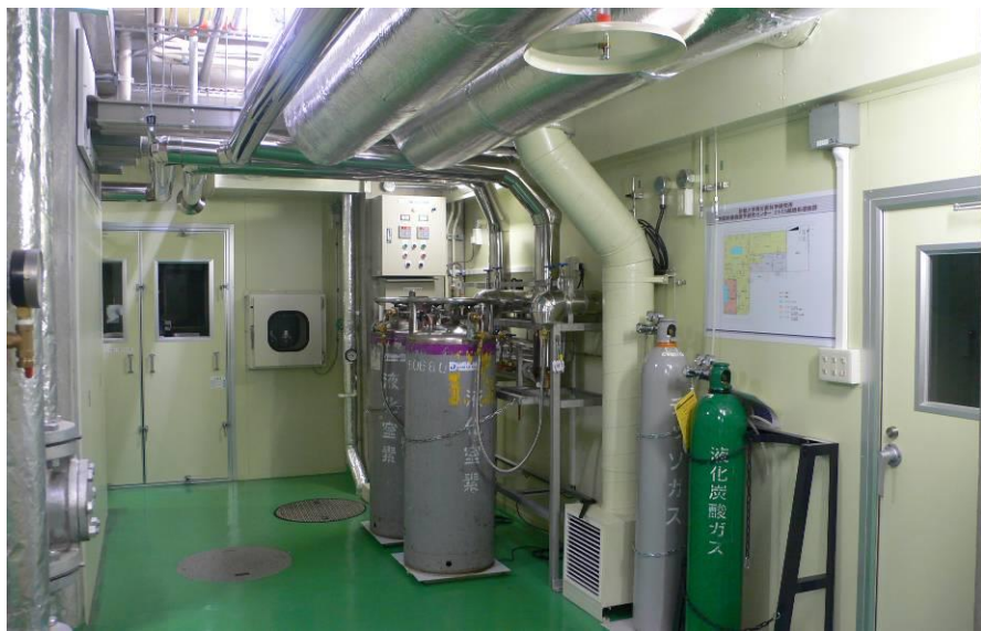
1. Entrance and Over view
